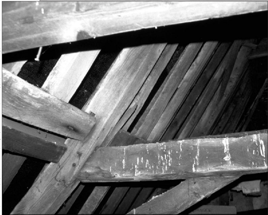
Roof beams in the Old White Lion, photo. 1988.
