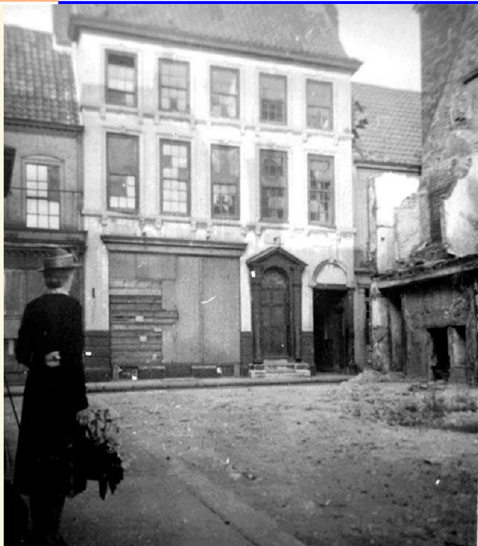
Photo. 31st July, 1947, by Philip Rumbelow (Lillian Rumbelow on left). Note that the house which was Dawson Turner's birthplace number 40 and 41 Middlegate is that depicted on Corbridge's plan. There is also a note about the house in Nall's Yarmouth, the large paper edition. These houses should have unquestionably been preserved and restored. Row 119 is to the left.
