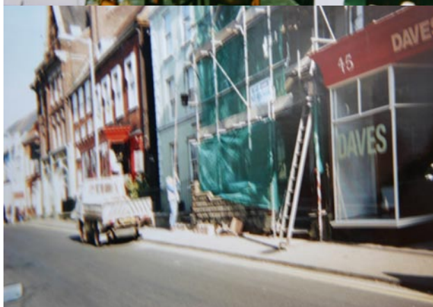
2.11.94, work in progress on 44 King Street. W. Wiseman, builders.
